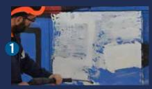
Clean the surface with pressurized water  $(\max 50 \, \text{bar})$ , for dirt removal. Warm water on metal surfaces helps in graffiti removal. The water temperature must not exceed  $80^{\circ}\text{C}$ . In the majority of cases most of the graffiti will be already removed with this step. If not, then follow the next step.
